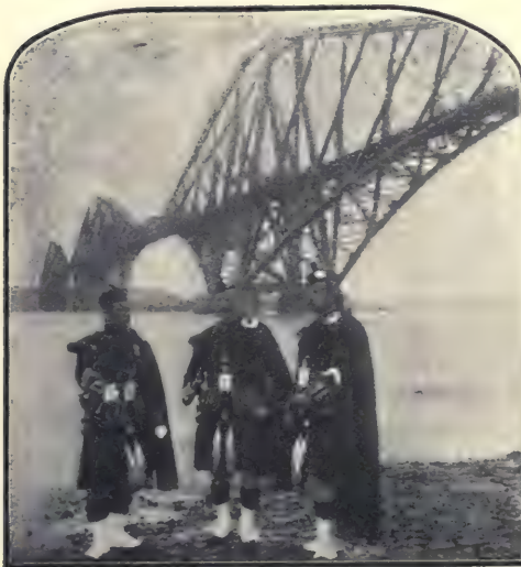
FIG. 211—The Great Forth Bridge, Scotland
